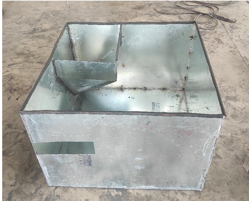
Fig. Fabrication of water storage tank
