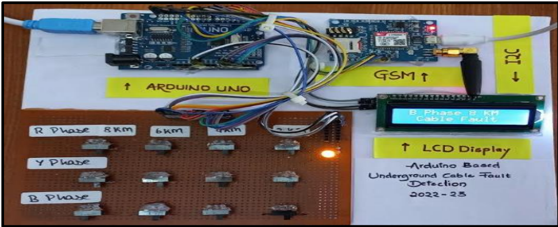
Figure 5 Cable Fault Detected at B-Phase ( 8Km Distance)
