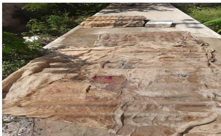
Figure (13) Curing of Precast segments
