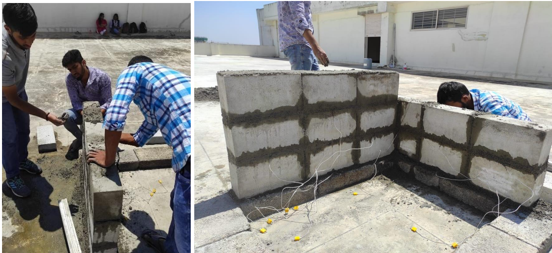
Figure 2.4 - Construction of wall with thermocouples implanted inside
