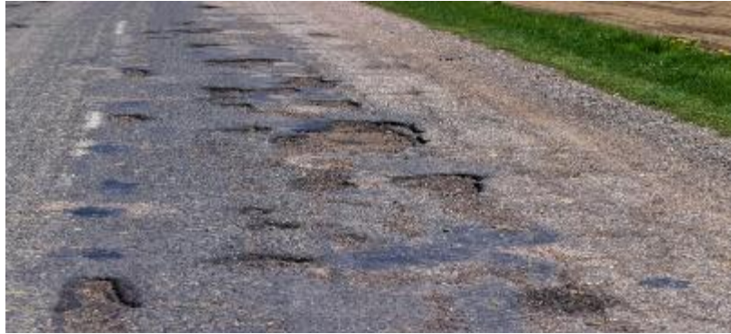
Fig.1.6: Types of Potholes
