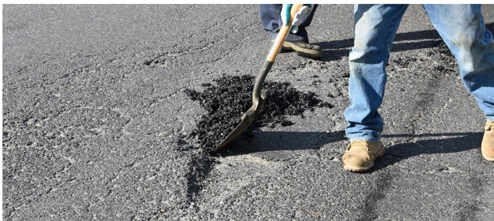
Fig. 1.7: Pothole Patching
