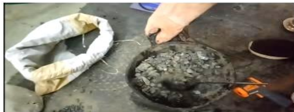
Fig.2 Mixing of aggregates with bitumen
