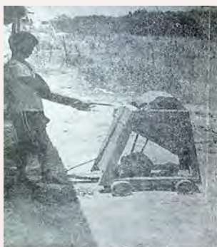
Fig 2. Sisal Decorticator in Operation
