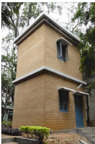
Figure 14. Demonstration building using IOT as fine aggregate.
